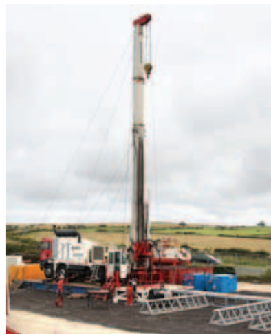
Drilling at York Potash
