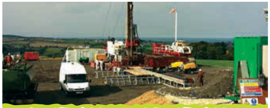
SM2 with coring rig on site – Autumn 2011.
